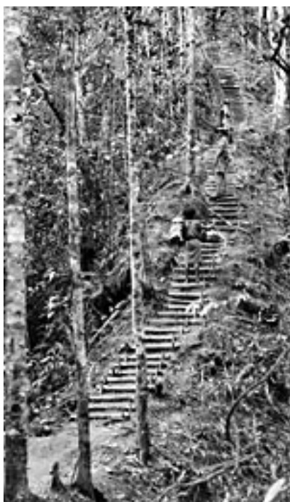
Figure 5: The ‘Golden Stairs’ rise towards Imita Ridge on the Kokoda Track, photographed in October 1942. [AWM 26837]
